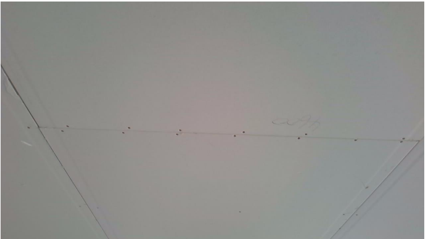
SHEETRS JOINED ON BLOCKING Taken at 10:23 AM on Wednesday 24/07/2024
