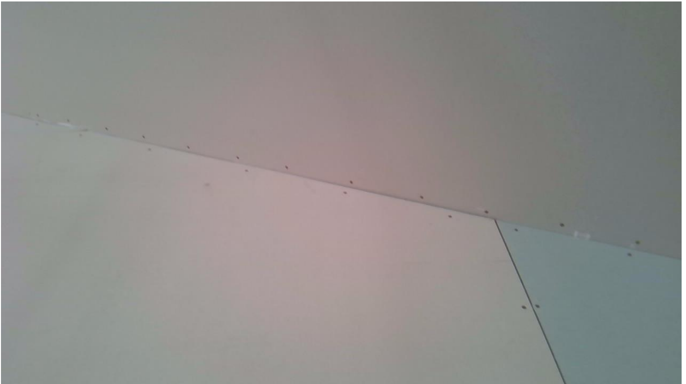
Spacing to be reduced from 150mm centres to 100mm centres Taken at 10:38 AM on Wednesday 24/07/2024
