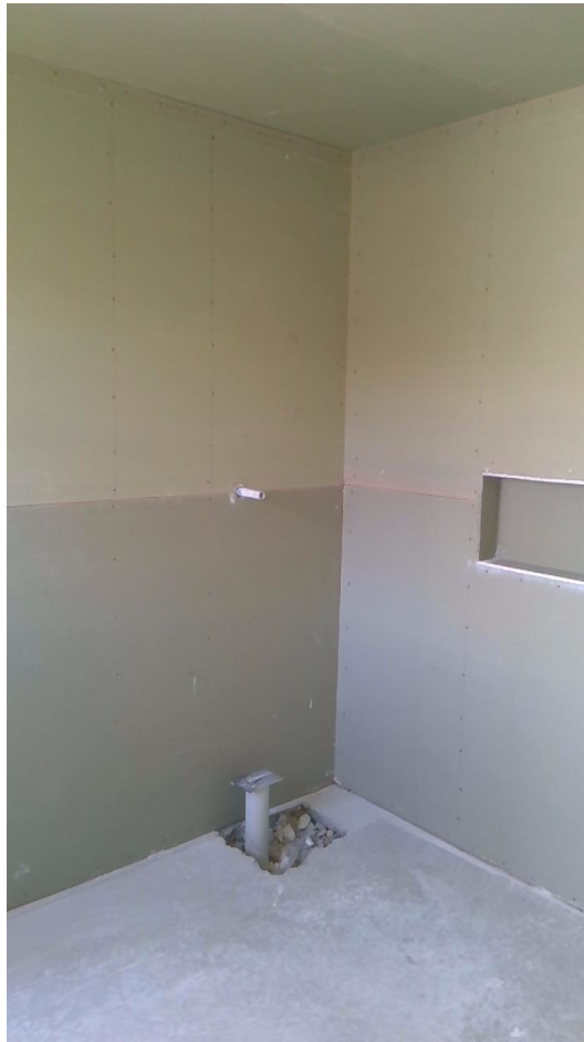
Ensuite tiled shower, no nogs behind the horizontal sheet joints Taken at 10:30 AM on Wednesday 24/07/2024
