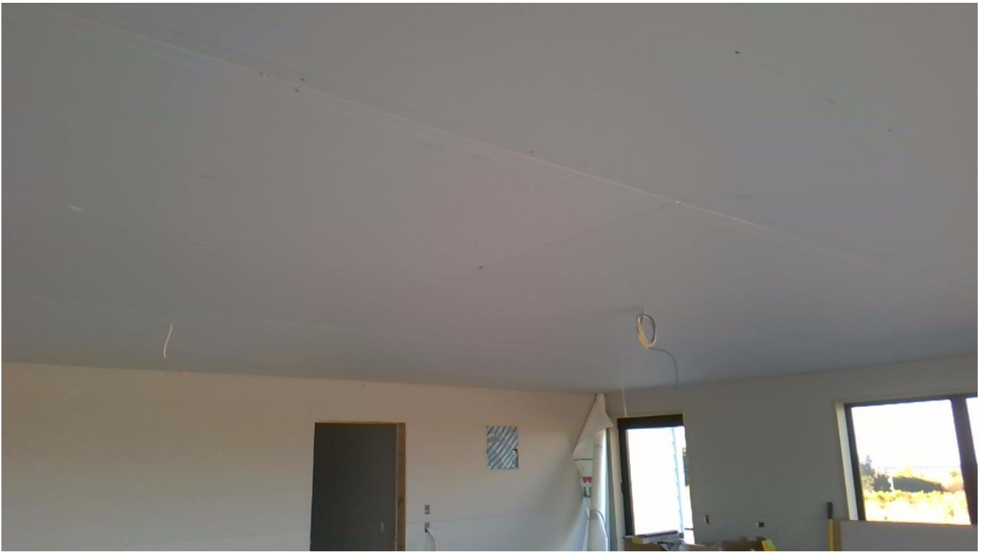
GARAGE DIAPHRAGM NO PENETRATIONS AT TIME OF INSPECTION ONLY CABLES Taken at 10:22 AM on Wednesday 24/07/2024
