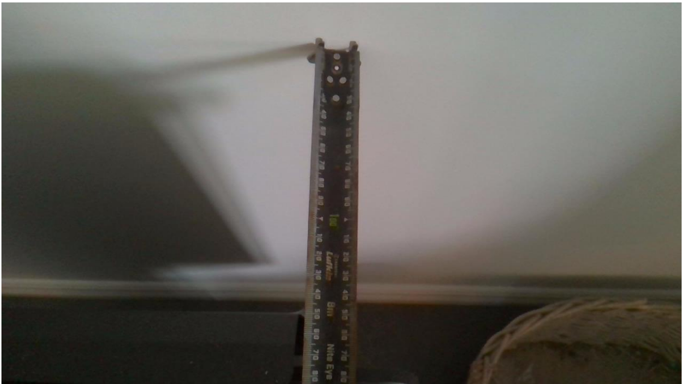
150mm rear wall clearance
