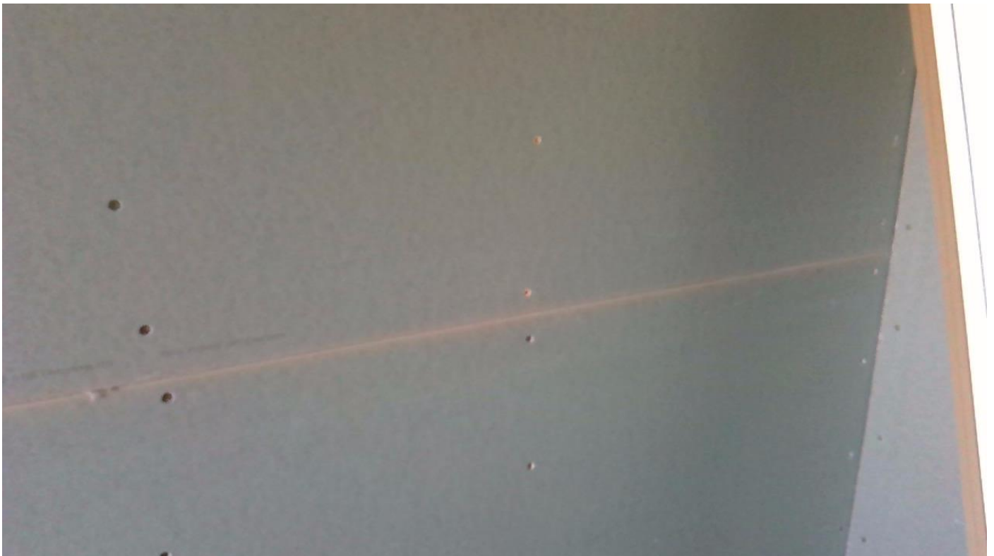
No nogs behind bathroom tiled shower side wall sheet joints Taken at 10:27 AM on Wednesday 24/07/2024
