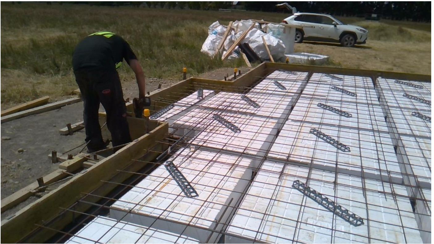
Corner bars being completed at time of inspection Taken at 1:33 PM on Monday 27/11/2023
