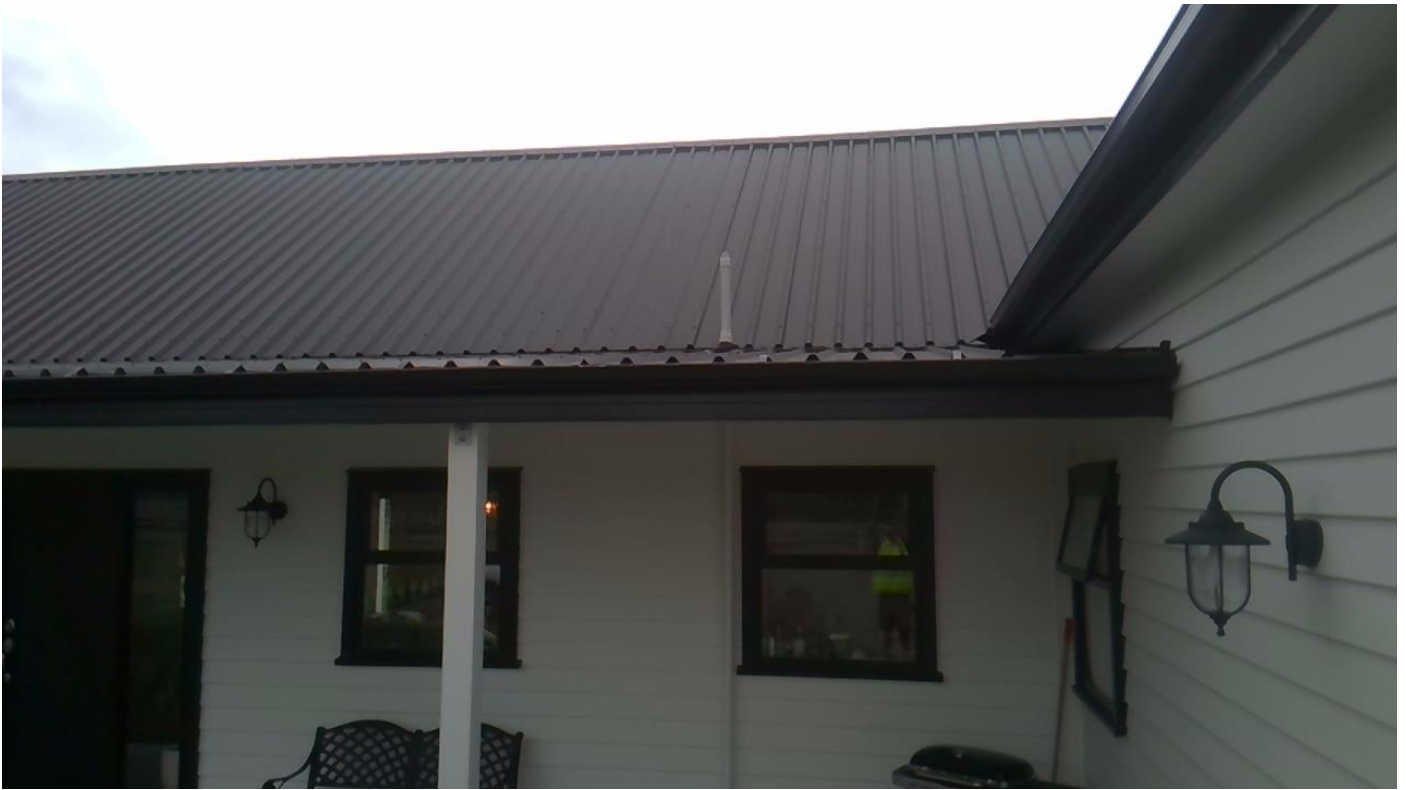
Branch vent in place, with dektite Taken at 10:49 AM on Friday 21/02/2025
